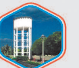
Water Tank 1 Lakh Ltr. Over Head
